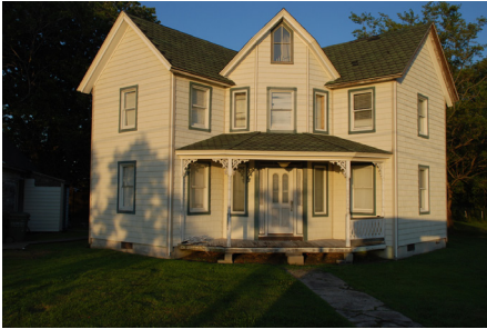
Figure 23 The "W" House is shaped to allow for air flow to be distributed throughout the house regardless of a breeze's direction - one of five remaining on Tilghman Island.
