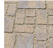
Figure 31 Permeable pavers applied to the turning radius
