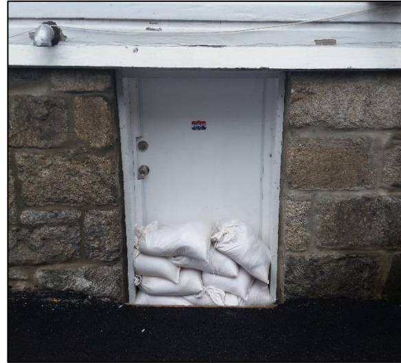
Photo 16: Sandbags installed at a below-grade entryway.
