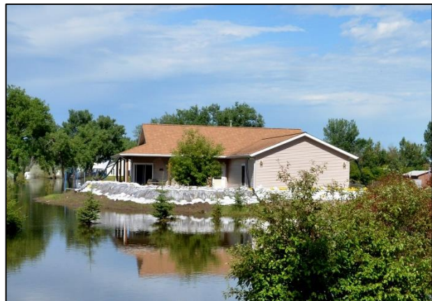
Photo 10: Sample of temporary earthen floodwall.
