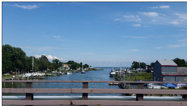
Photo 18: View from Tilghman Island Drawbridge.
