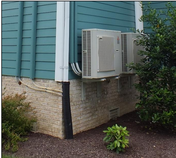
Photo 13: Sample of elevated utilities mounted to the building.
