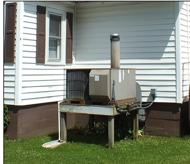
Photo 14: Sample of elevated utilities on a platform.
